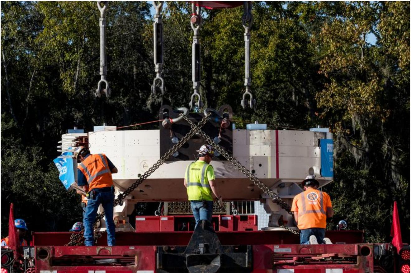
Construction workers connect a part of the cyclotron to the crane so that it can be lowered into the building at Provision CARES Proton Therapy Center at Horizon West. (Sarah Espedido / Orlando Sentinel)
